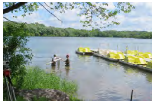
Staff install a water level sensor on Hyland Lake. The sensor tracks how high the lake gets.
