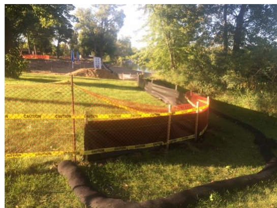
Temporary and permanent erosion control measures are essential to reducing pollution in runoff
