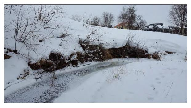
Figure 5-4 Erosion upstream of crossing with Lake Riley Road
