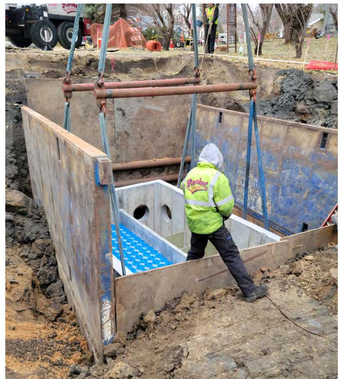
Kraken® filters were installed in November 2021.
