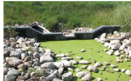
Example of a stage weir from the *Minnesota Wetland Restoration Guide* by the Minnesota Board of Water and Soil Resources (BWSR)
