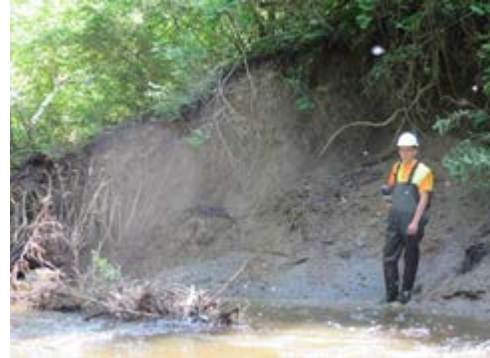
A severe bank erosion site in the Lower Valley as observed in 2014.
