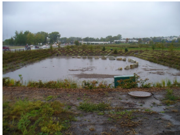
Iron-enhanced sand filtration system near Beam Avenue following a rainfall event.
