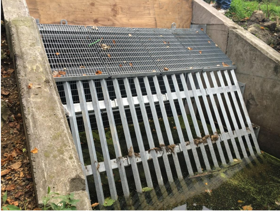
Figure 10. Carp barrier below PCCA. The barrier (metal grid) is placed behind a debris rack located upstream.
