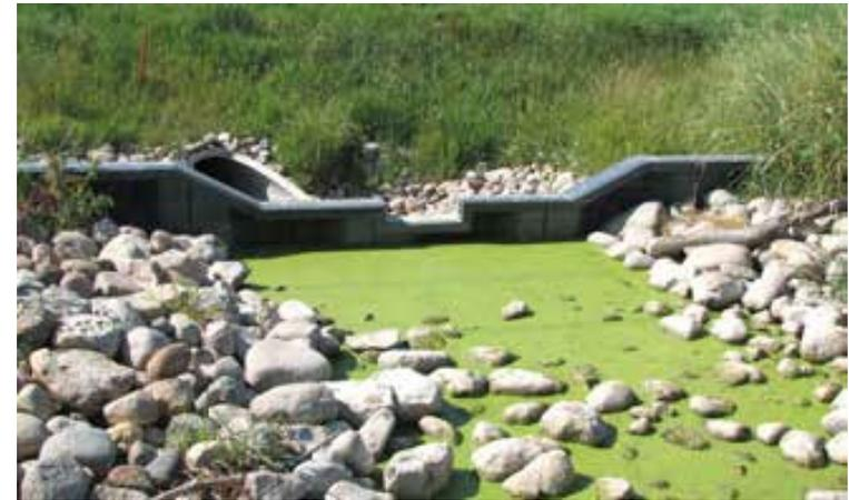
Example of a stage weir from the *Minnesota Wetland Restoration Guide* by the Minnesota Board of Water and Soil Resources (BWSR)
