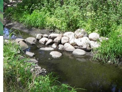
**Cross Vanes** control stream bed elevations, dissipate flows, provide pool habitat
