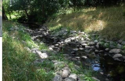
**Rock Riffles** create natural channel patterns, control stream bed elevations, provide habitat diversity
