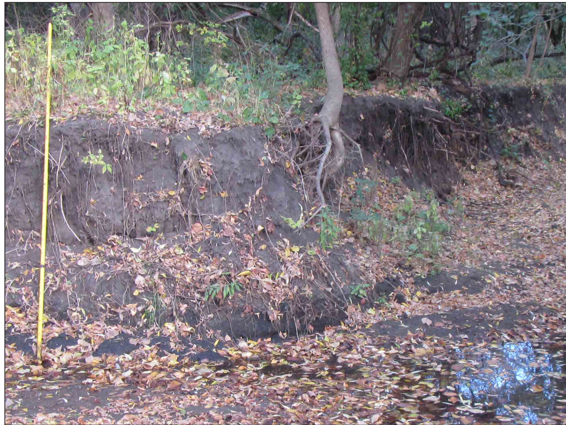
Steeply eroded streambank
