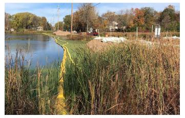
A double row of yellow silt curtains in the water protect the lake from the Duck Lake Road construction zone (fall 2021).
