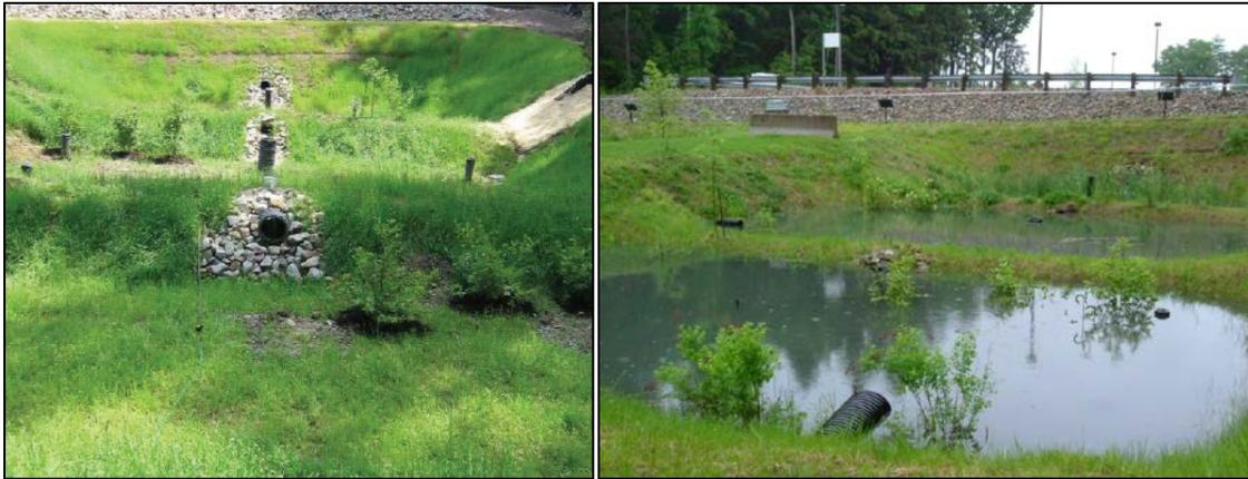
Subsurface gravel bed wetland used in the UNHSC study on the BMP's treatment effectiveness. Image on left shows the basin during dry weather conditions. Image on the right shows the basin during a rain storm (University of New Hampshire Stormwater Center, 2010).
