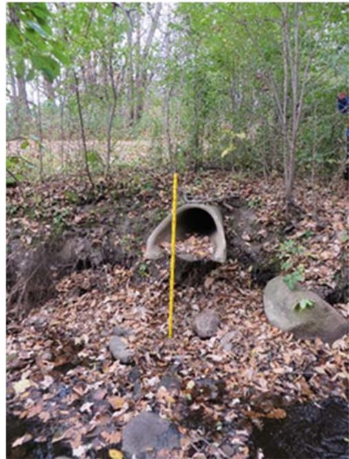
Photo 9-2 Suspended stormwater culvert in sub-reach P7E
