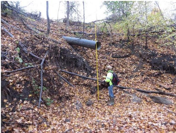
**Photo 7-1 Suspended stormwater culvert with large eroding bank**
