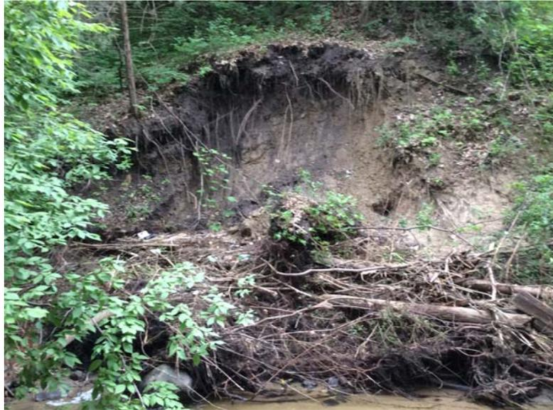
Photo 1-1 Eroding bank downstream of Culvert
