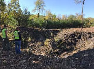
Cleared area of Bluff Creek Tributary (channel is approximately 10-12 feet deep). Litter from clearing was left on the ground to act as mulch for erosion control.
