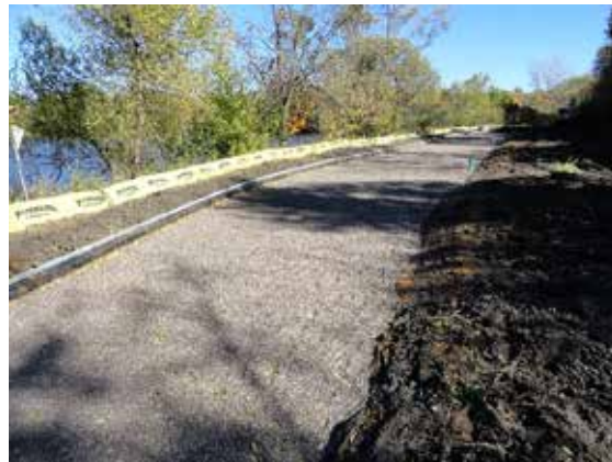
Photo of the completed water iron-enhanced sand filter, pre-restoration
