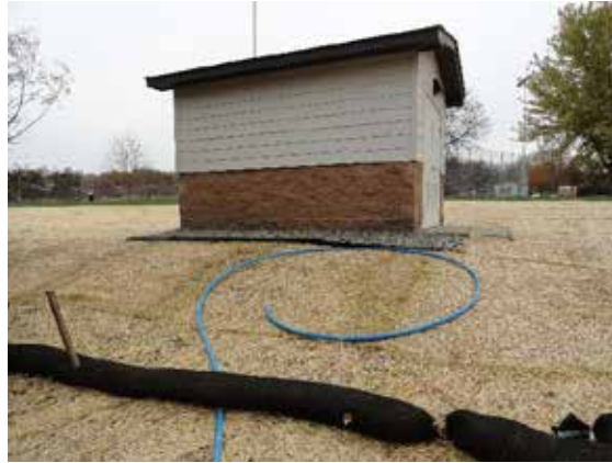
Photo of the completed water treatment shelter and blanketed area surrounding
