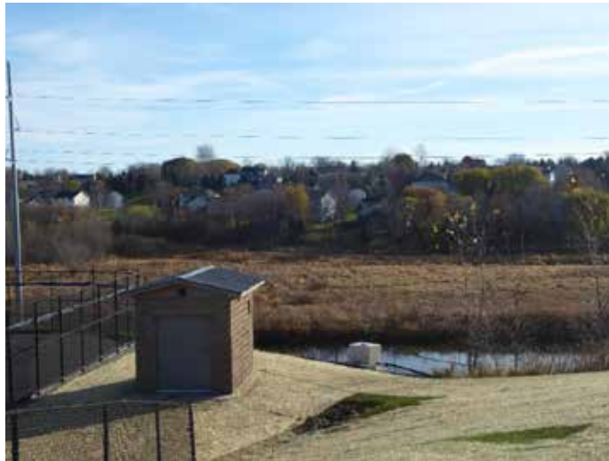
Photo: Treatment Shelter, Pump System, and Stormwater Pond (after site restoration). 10/31/2018
